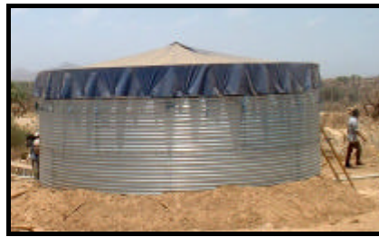
The 95,000 litre balancing reservoir
