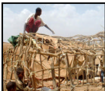
ICRC tents provide temporary shelter.
