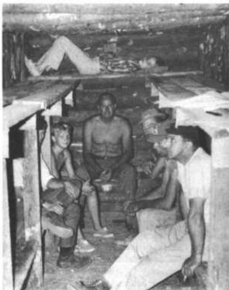
Benches with overhead wooden bunks are shown in Fig. 14.2. These were installed in a Small- Pole Shelter 6 feet wide with a ceiling almost 7 feet high.
