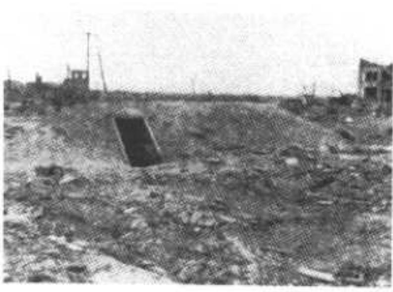
Although the shelter itself was undamaged, its occupants would have been fatally injured because the shelter had no blast door. The combined effect of blast waves, excessive pressure, blast wind, and burns from extremely hot dust blown into the shelter (the popcorning effect) and from the heated air would have killed the occupants. For people to survive in areas of severe blast, their shelters must have strong blast doors.
