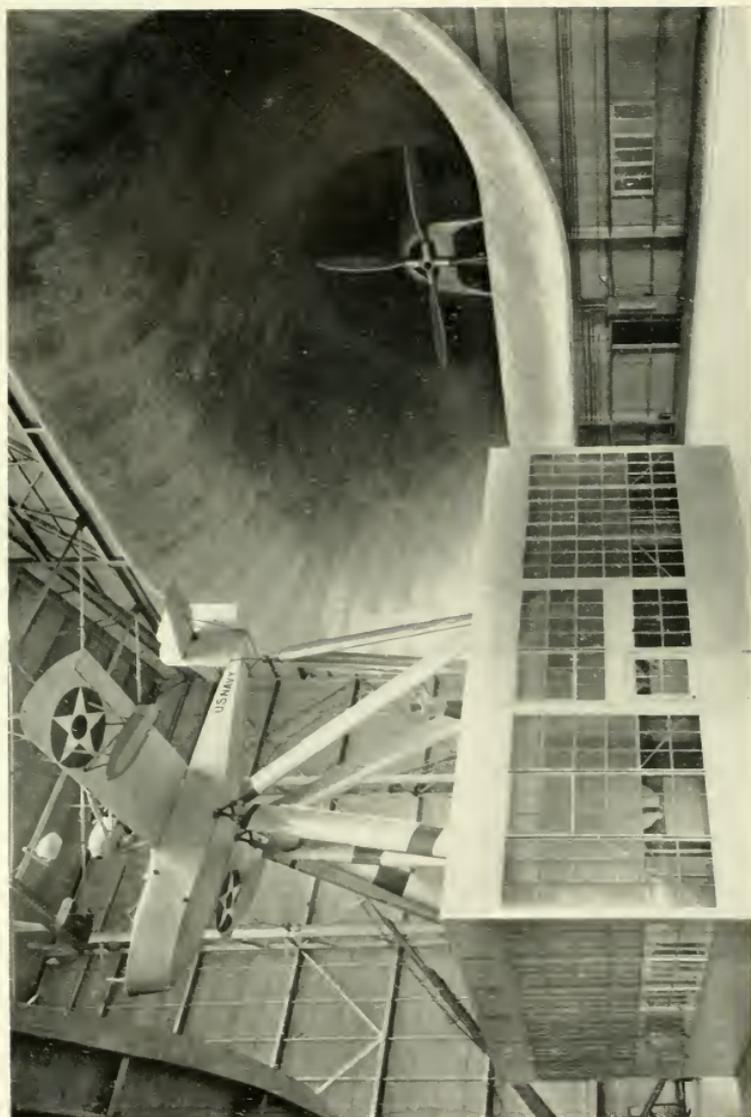
N.A.C.A. full-scale wind tunnel. View showing scaplane on balance and one of the 35½-foot propellers.
