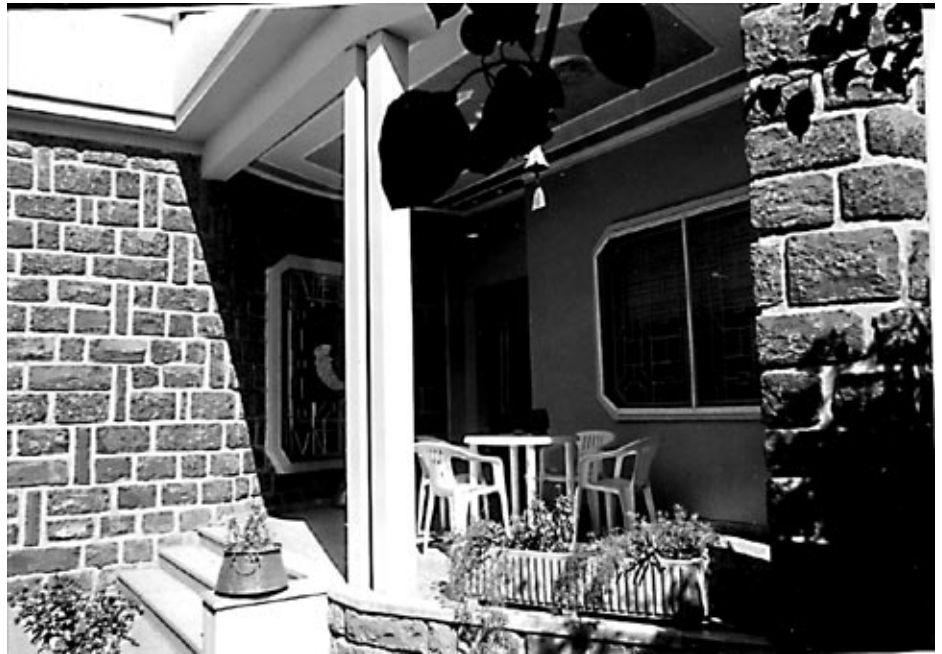
one of the houses the American Embassy leases in Asmara
